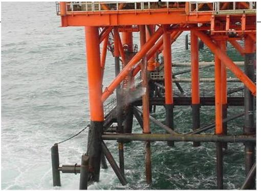
The Caisson had several clamps fitted to provide integrity, however leakage was still occurring below the clamps
