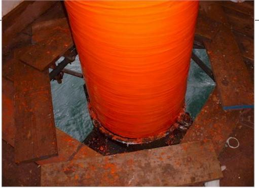
Two coats of IMG Offshore's one pack epoxy paint, Liquid Armour, were applied to match the existing platform colouring - Safety Orange
