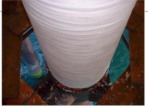
The Composite was compressed into place over 360 degrees using the IMG Offshore Uniwrap compression system
