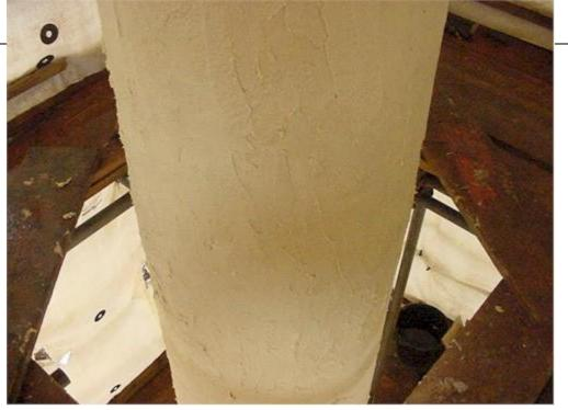
Once cleaned, IMG Offshore's Reinforced Epoxy was applied, at a 3mm rate over the 15 metre. A fibre support sheet was embedded into the epoxy.
