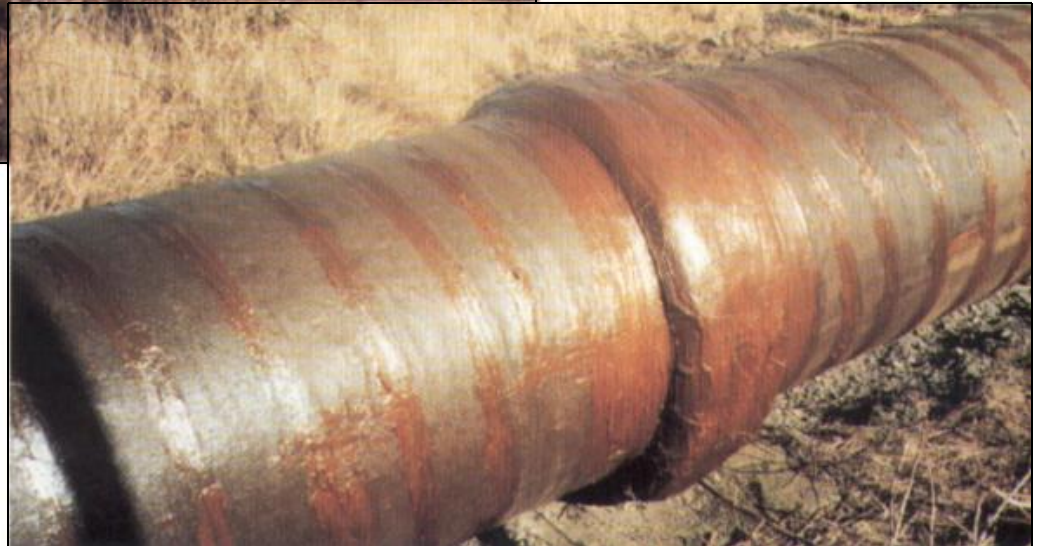
Northumbrian Water, Teeside: Refurbishment of Conduit 58
